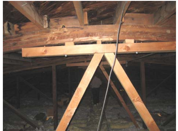
Fig 2- Repaired Roof Truss Area 2
